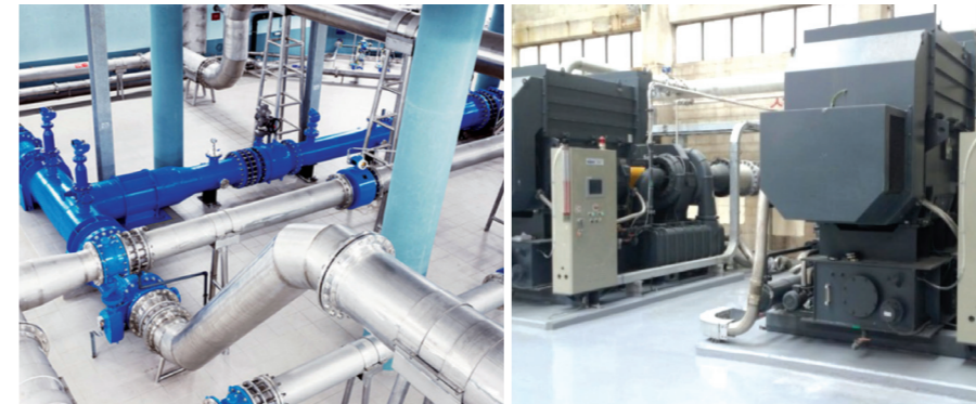
Machinery Construction Work
