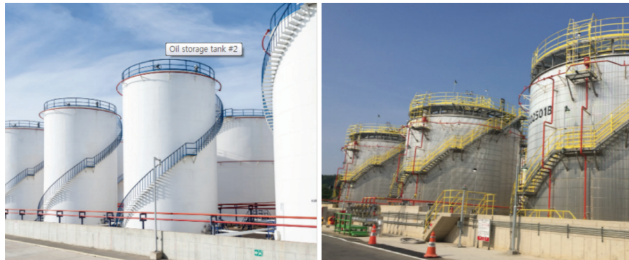
Tank Terminal & Steel Structure Construction Work
