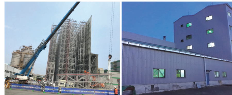
Plant & Structure Dismantling Work
