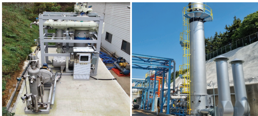
Environmental Construction Work (Atmospheric)
